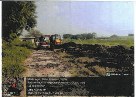
Fly Ash disposal site in Village Sikri Kalan, Modinagar, Ghaziabad.
